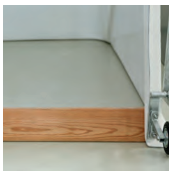
Threshold at the hut entrance stops bedding getting out
