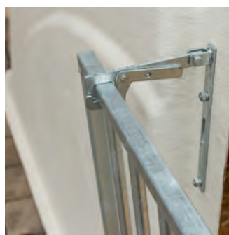
Side guards stop calves from slipping through and lend stability
