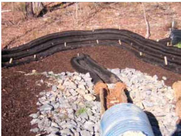
Figure 2 Compost filter socks used for capturing sediment
