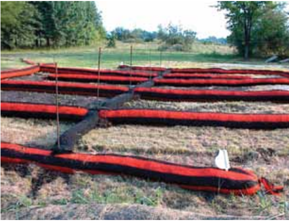
Figure 5 Compost filter sock biofiltration system
