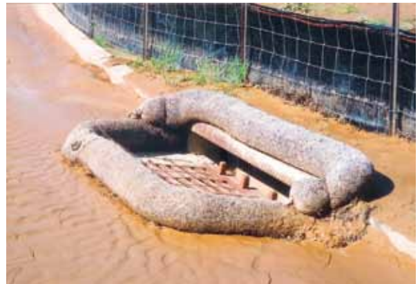
Figure 4 Compost filter sock curb inlet
